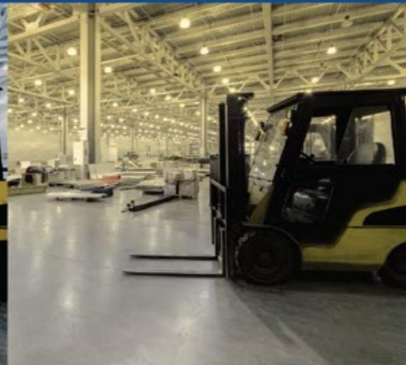
High-pressure sodium's produce a yellow light and is often referred to as "dingy light." It is hard to distinguish colors underneath this lighting.
